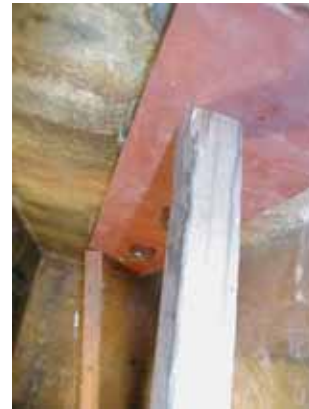
ARG installation surface (bottom view)
