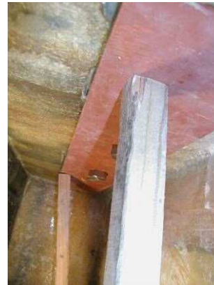
ARG installation surface (bottom view)
