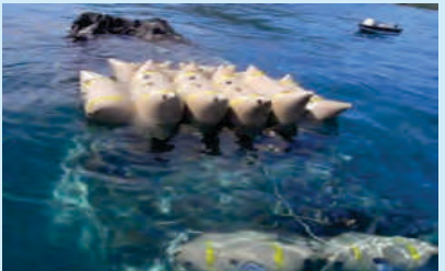
Shallow water wreck removal using clusters of Enclosed Flotation Bags 2,000 lbs.
