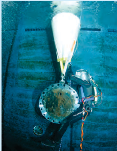
Commercial Lift Bag replacing a flange plate at the Atlanta Aquarium.
