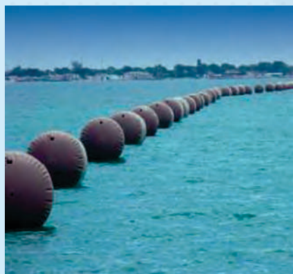
SP-6000's used to support a pipeline during installation.
