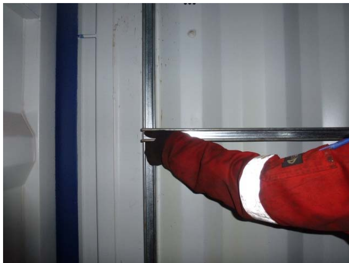
Showing Unistrut and demonstrating how a thumb could become trapped within it
